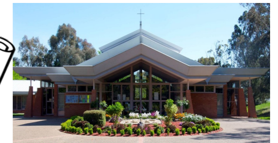
St Michael's Church Tyrrell Cct Kaleen
